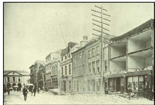
Damage resulting from the 1886 Charleston earthquake. More than 60 persons were killed.
