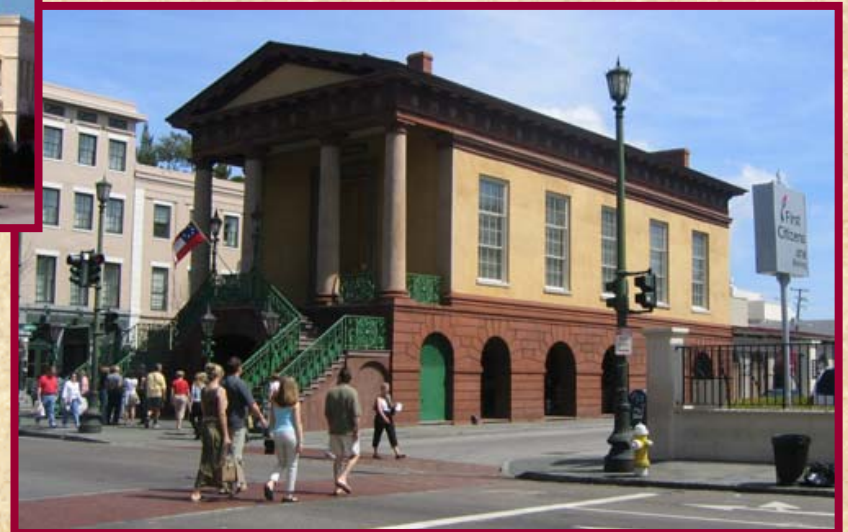
Market Hall Charleston, S.C. 1841
